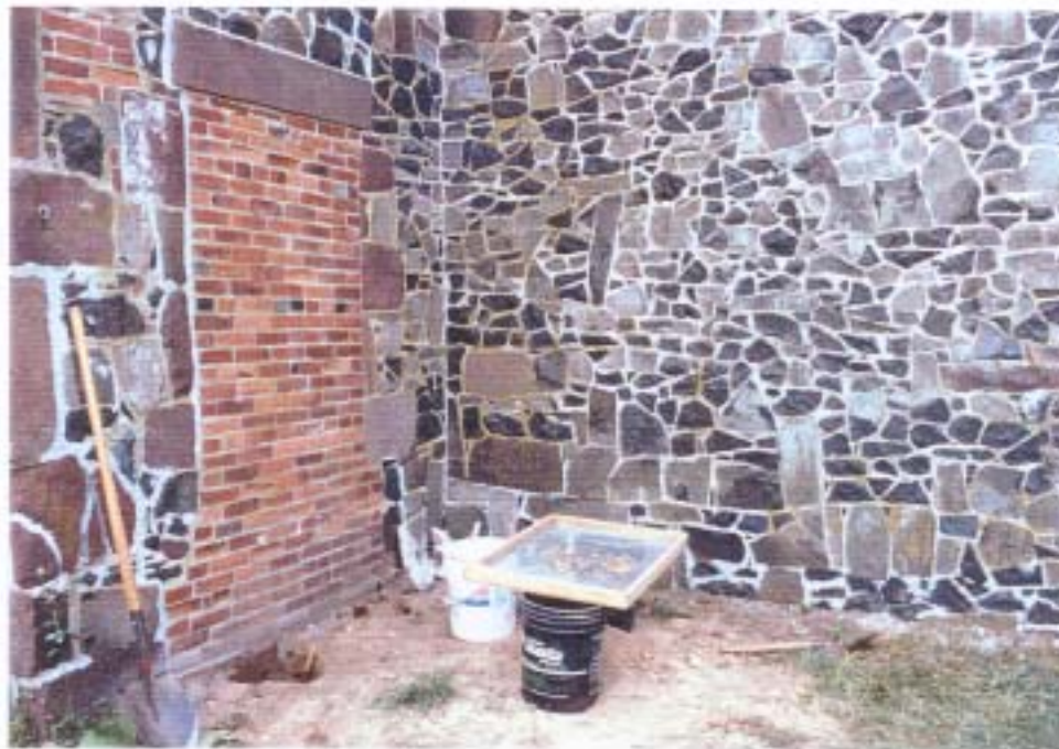
PHOTO 8 - THE NORTHWEST CORNER ----- OF THE HOUSE -----
